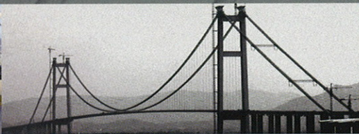
Ruyang Suspension Bridge
